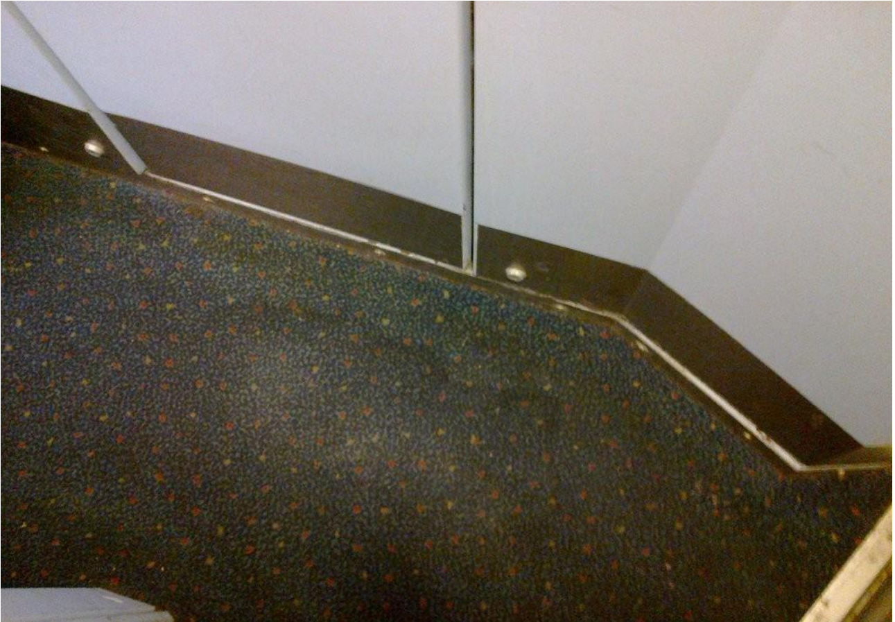
Urine-soaked carpet from overflowing toilet
