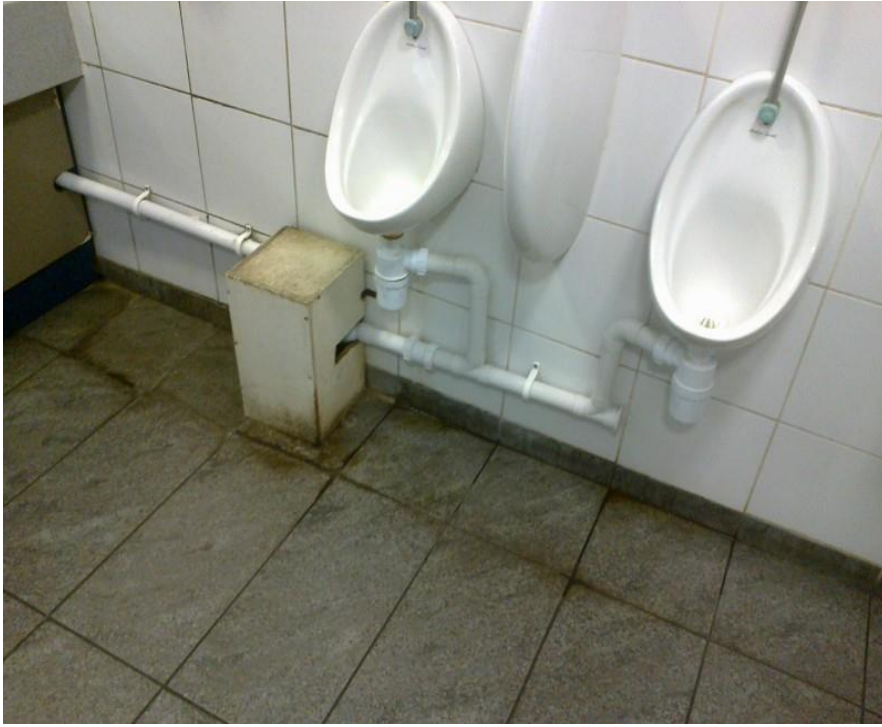
Leaking toilets at Woking and Basingstoke
